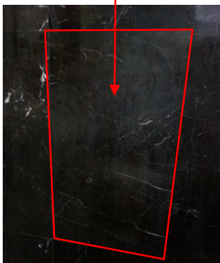
Streaks mark on bathroom marble wall
